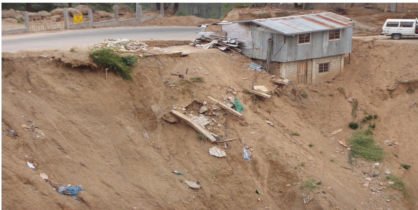
Landslide damage. Photo: International Disaster Volunteers / Flickr
